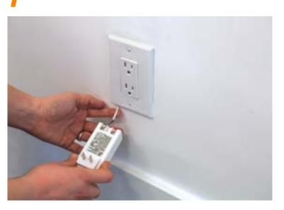
Gently pull the power wire through the wall at the outlet end. You may need to remove your outlet cover to do this.
