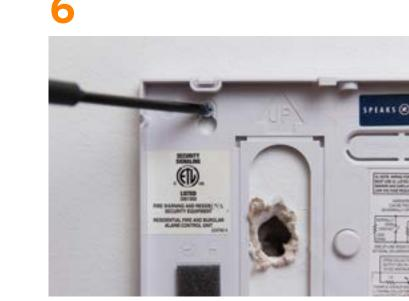
Remove the screws from the backplate of your panel and remove the panel from the wall. Please note there will be a small hole in the wall.
