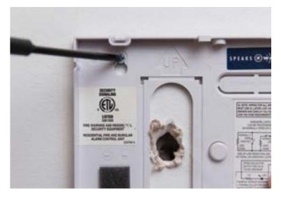
Remove the screws from the backplate of your panel and remove the panel from the wall. Please note there will be a small hole in the wall. 7
